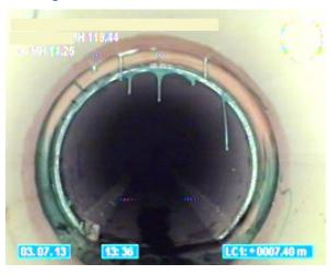
**Figure 11 Excessive Solvent Cement**
